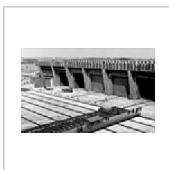
Bau des U-Boot-Bunkers in Lorient , April 1942
